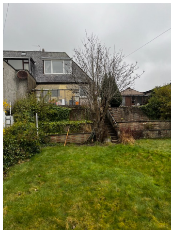
Rear view, house sits at a higher level than the rear garden allowing for basement area.
