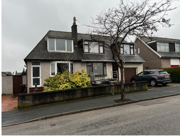
View of appeal site No.21 Balgownie Crescent and adjoining house at 23 Balgownie Crescent, previously extended to front and rear.
